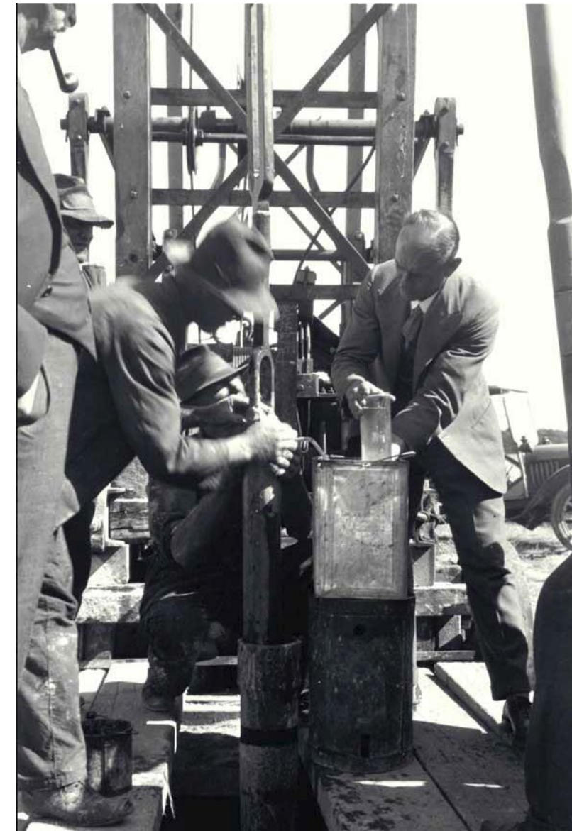
Collecting gas from the Ramsay Oil Bore 1 near Minlaton in 1931. The well reached ~550m, and a small gas flow of almost pure hydrogen was recorded.
