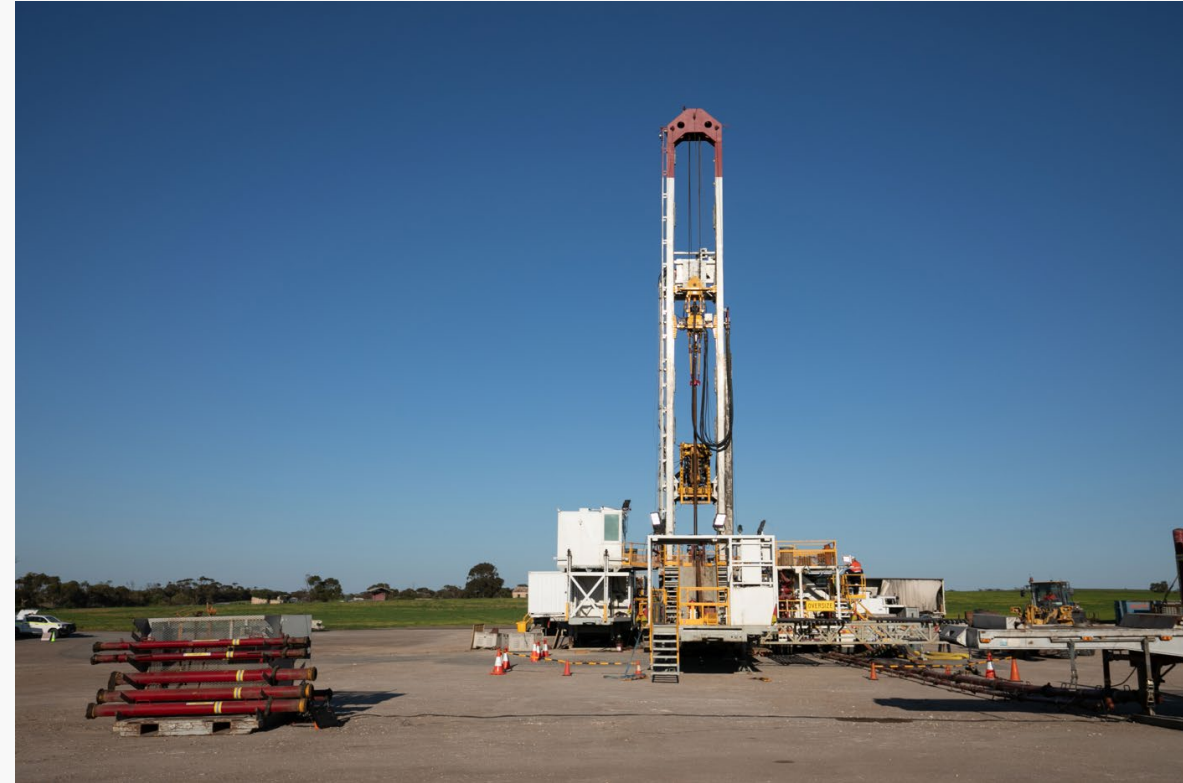
Ramsay 1 drill site and Savanna Energy drill rig
